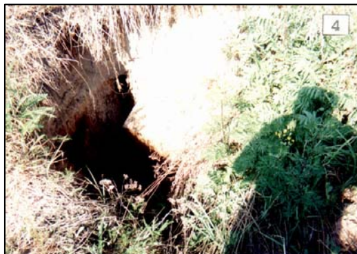
KOMPLEKSNY – VAULT AND PIT THROUGH CLAY CAP
